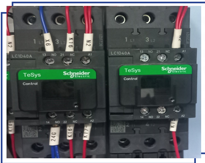
Brand: Schneider Electric TeSys (x2) Model: LC1D40A Power: 3PH 415V 40A 22kW 50Hz
