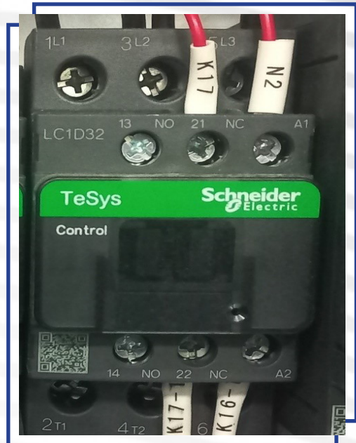
Brand: Schneider Electric TeSys Model: LC1D32 Power: 3PH 400V-415V AC 32A 15kW 50Hz
