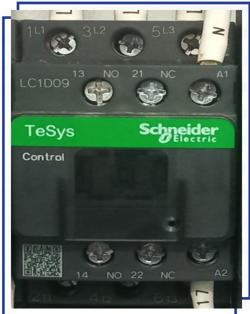
Brand: Schneider Electric TeSys Model: LC1D09 Power: 3PH 380V-400V AC 9A 50Hz
