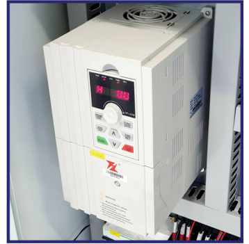
Fuling Inverter 7.5kW
