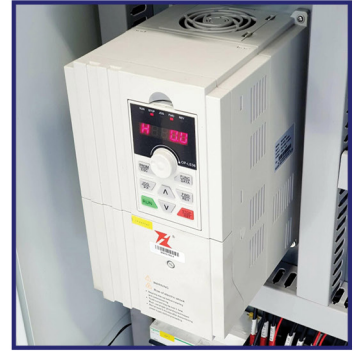
Fuling Inverter 7.5kW
